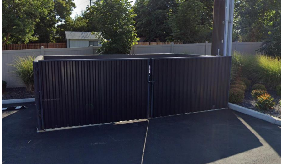
Typical WTB trash enclosure
