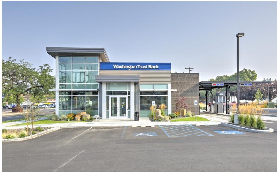
Example of site lighting in another WTB project
